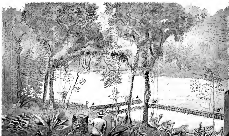
A CAISSON ABOUT COMPLETED.
